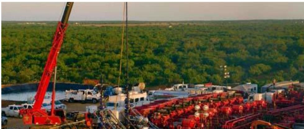
By utilizing zipper fracking, Swift Energy can hydraulically fracture multiple wells in less time, increasing the number of fracking stages completed per month.
