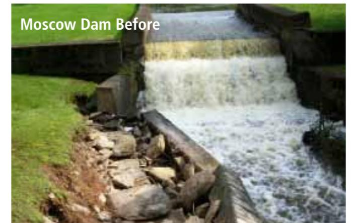
collaborated with Gannett Fleming, Inc., to develop an innovative and environmentally friendly solution to restore a stream at Valley Forge National Park and protect a major transmission main exposed by erosion over a 55-year period.
