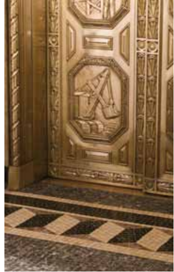
595 Madison Avenue Historic Elevator Doors
