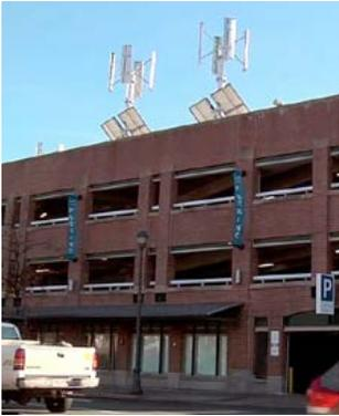
*Verizon teamed up with Wing Power Energy to erect small wind/solar turbines on the roof of our building in Salem, Mass.*
